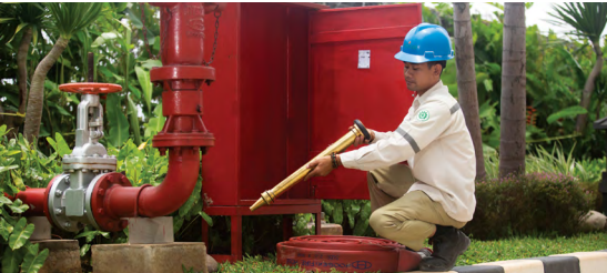
An employee conducting routine inspection of fire safety equipment
